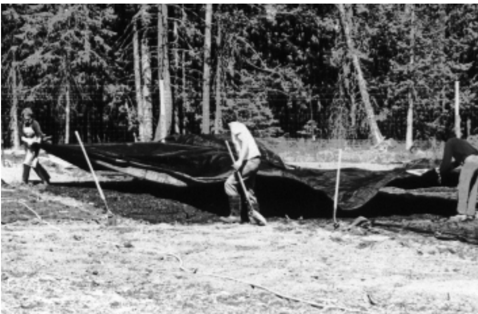
Figure 3. Covering the ground with plastic.
